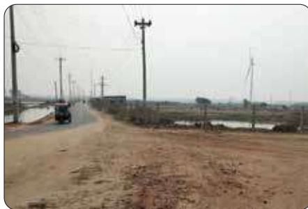
Figure: 60 MW US-DK Wind Power Plant, Khurushkul
